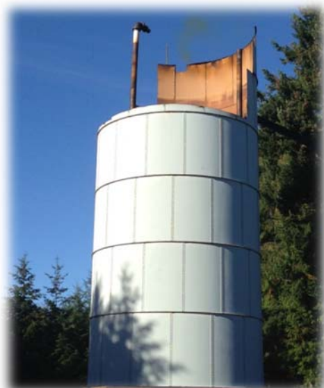
Beachcomber Reservoir Demolition 2015
