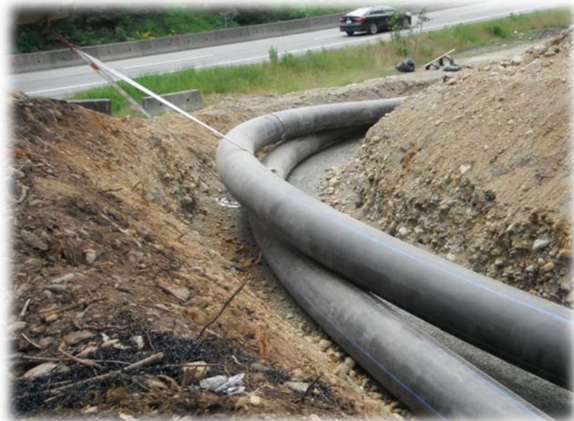
Bulk Water Transmission Line Construction near Hwy 19 (2017)
