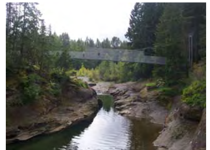
Top Bridge Crossing - a key link in the regional trail network.
