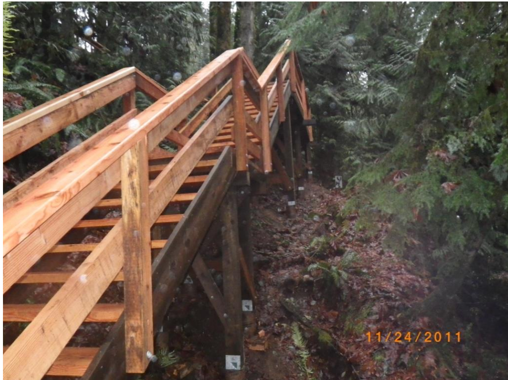
Figure 16. Stairs installed in steep, sensitive terrain within Stocking Creek Regional Park, in the Cowichan Valley Regional District park system.
