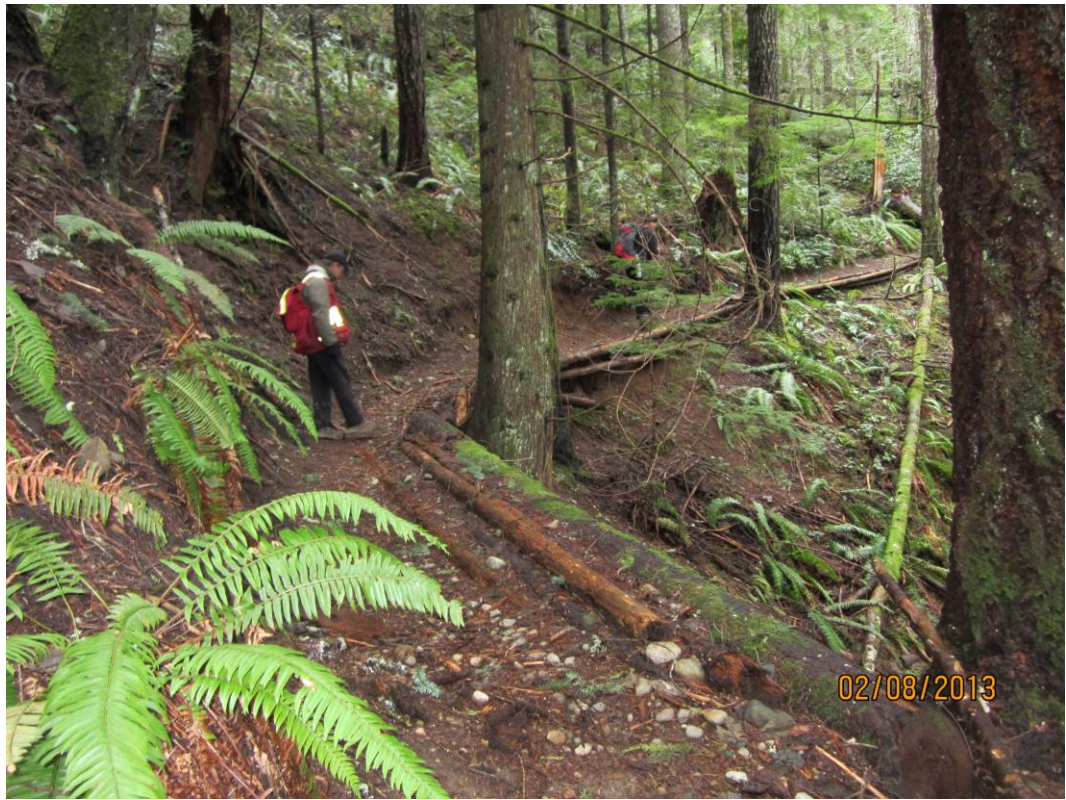
Figure 17. Small diameter logs are used to stabilize and delineate trails adjacent to BCFRP.
