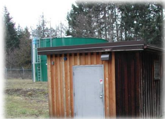
French Creek Main Pumphouse and Reservoir
