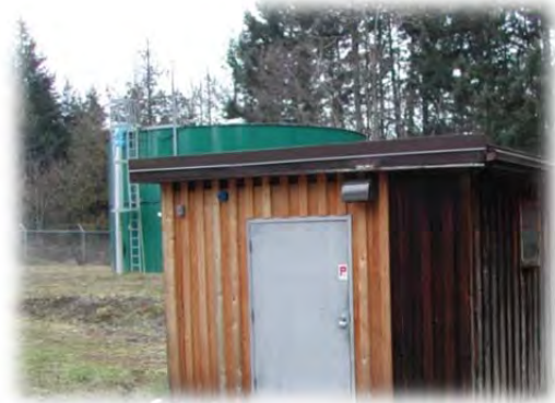
French Creek Main Pump House and Reservoir
