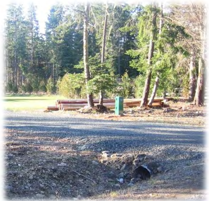
Watering Sampling Station on Rascal Lane
