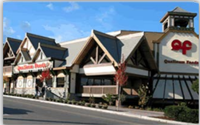
Example of different materials and colours used in combination to create contrast and to reduce massing of a prominent building in the Qualicum Beach village center.
