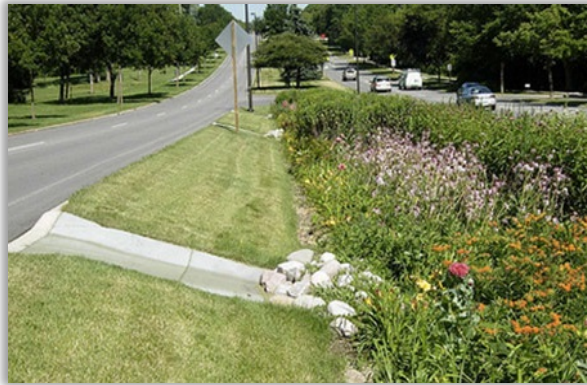
Examples of a rain garden and rainwater harvesting system.
