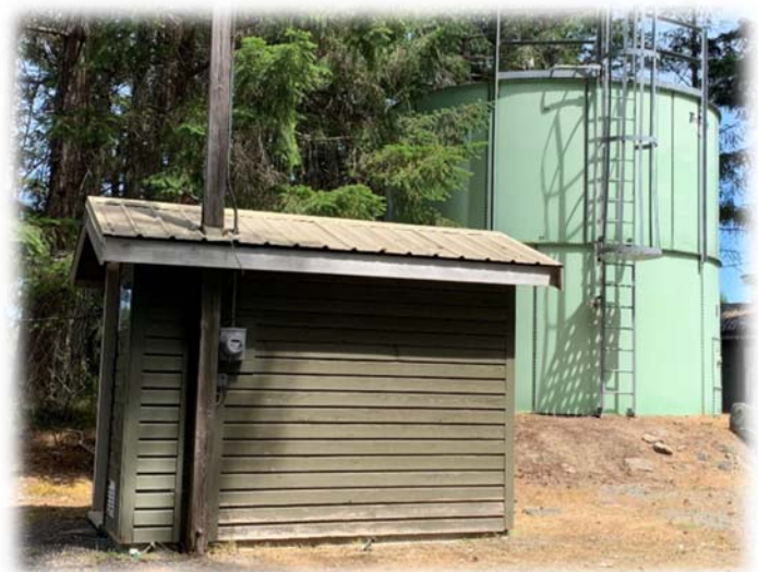
Decourcey Pumphouse and Water Storage Reservoir
