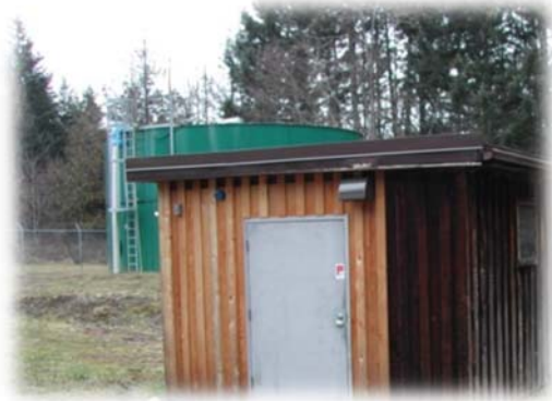
French Creek Main Pump House and Reservoir
