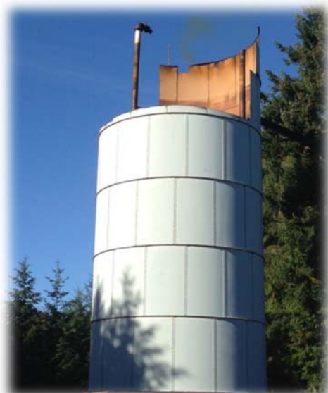
Beachcomber Reservoir Demolition 2015
