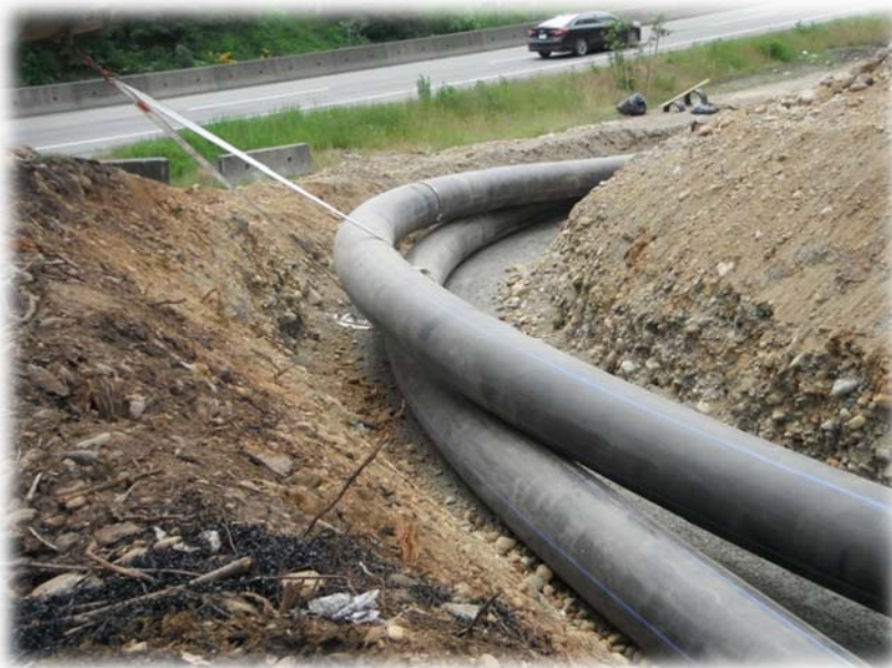
ERWS Bulk Water Transmission Line Construction near Hwy 19 (2018)
