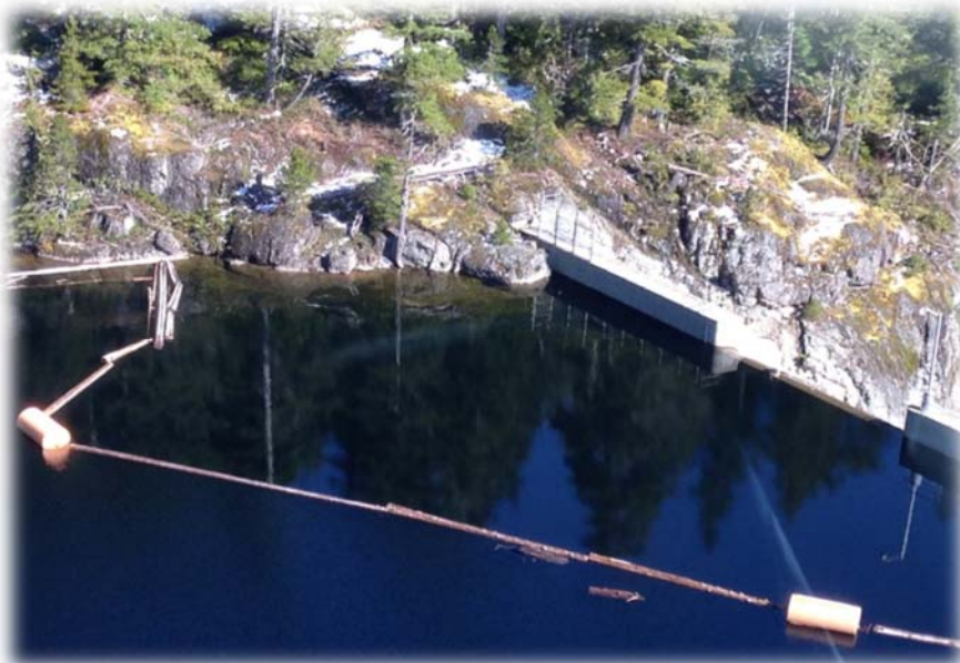
Arrowsmith Dam April 2014
