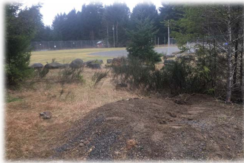
Rollo McClay Wellhead Decommissioned
