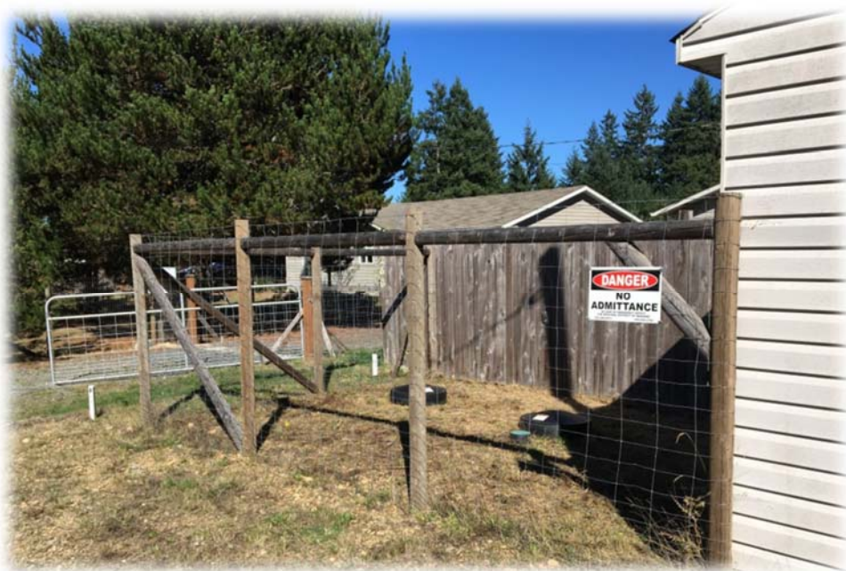
Well site and fence
