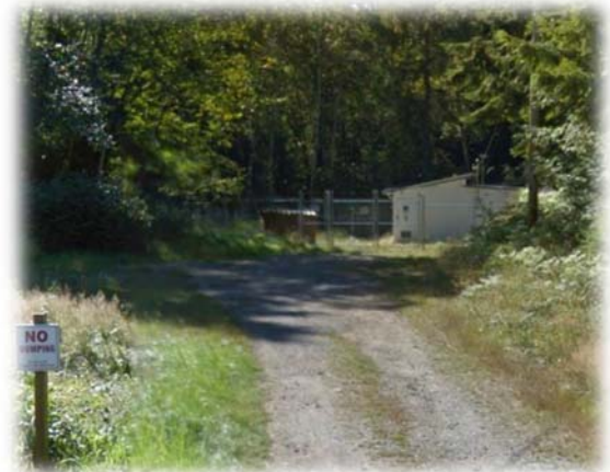
Water Intake Location and Pumphouse
