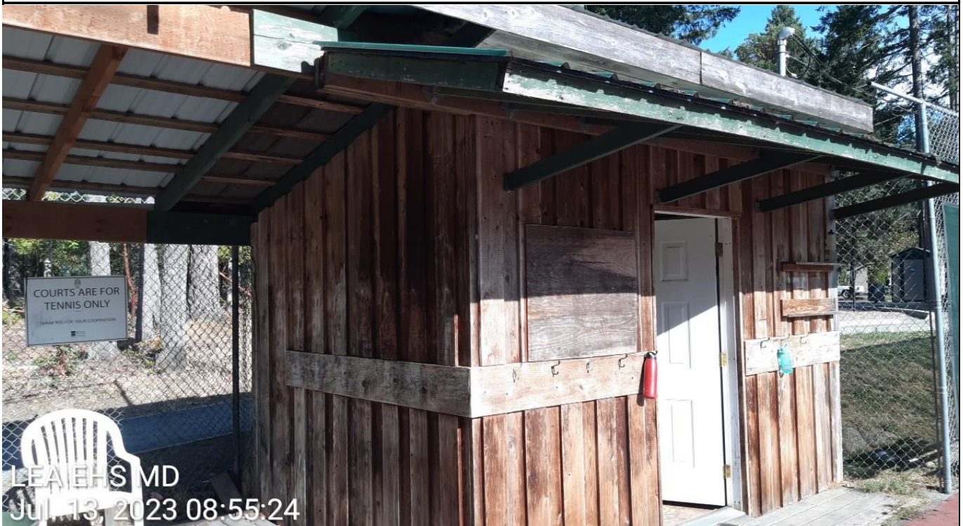
Figure 2. Exterior of Building Showing Wood Siding and Sheet Metal Roofing
