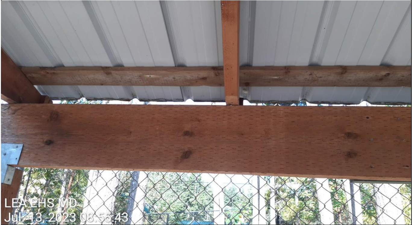
Figure 1. Pressure Treated Lumber on Exterior Posts/Framing
