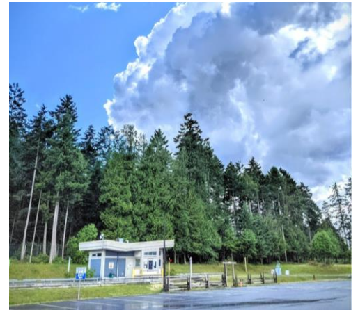
Church Road Transfer Station – Scale House
