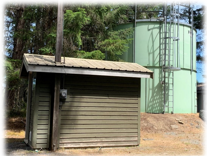
Decourcey Pump House and Water Storage Reservoir
