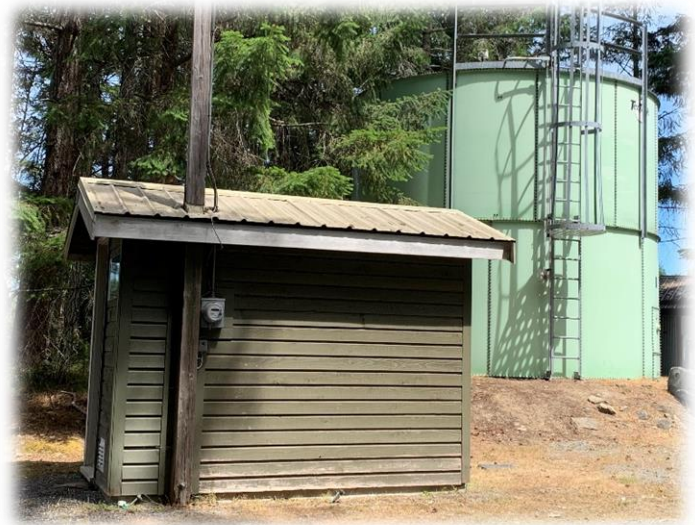
Decourcey Pumphouse and Water Storage Reservoir
