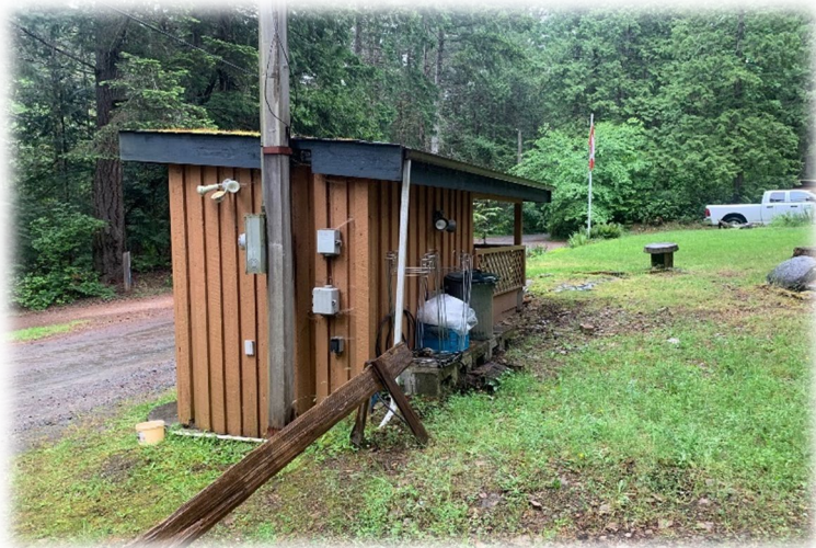
Descanso Bay Park Treatment Building
