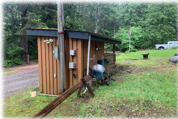
Descanso Bay Park Water Treatment Building
