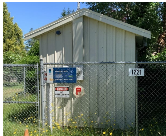
French Creek Well #2 pumphouse
