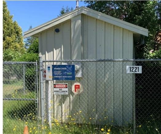
French Creek Well #2 pumphouse
