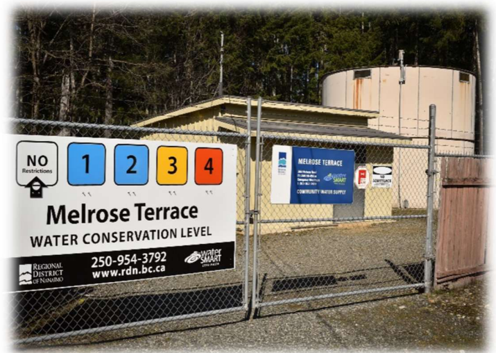
Melrose Pumphouse and Reservoir
