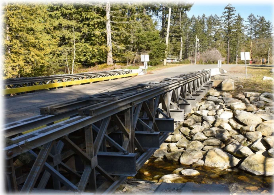
Melrose Road Bridge
