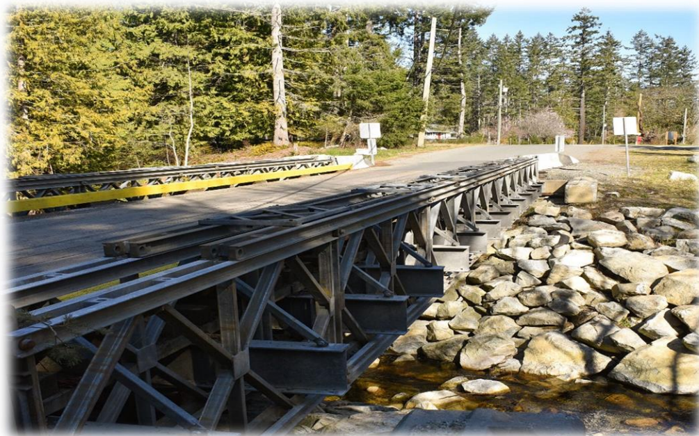
Melrose Road Bridge
