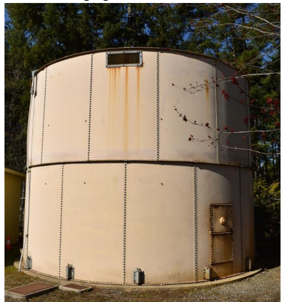
Melrose Water Storage Reservoir
