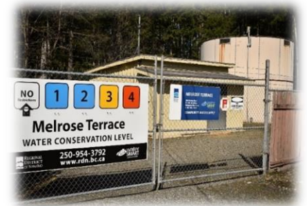
Melrose Pumphouse and Reservoir
