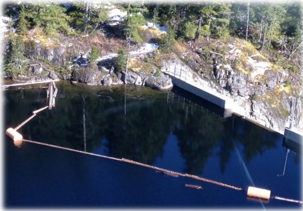
Arrowsmith Dam April 2014
