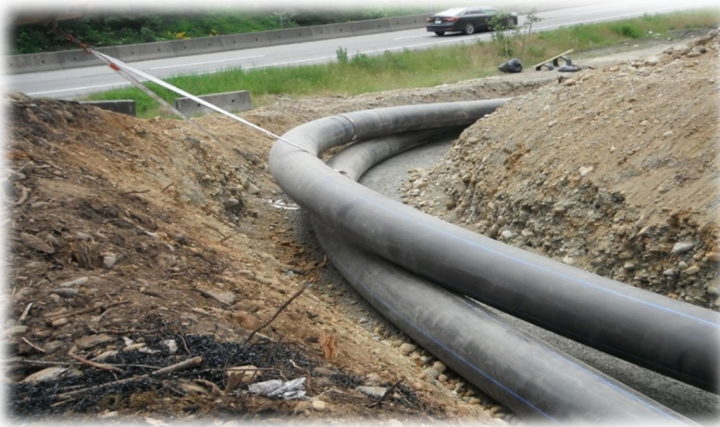
ERWS Bulk Water Transmission Line Construction near Hwy 19 (2018)
