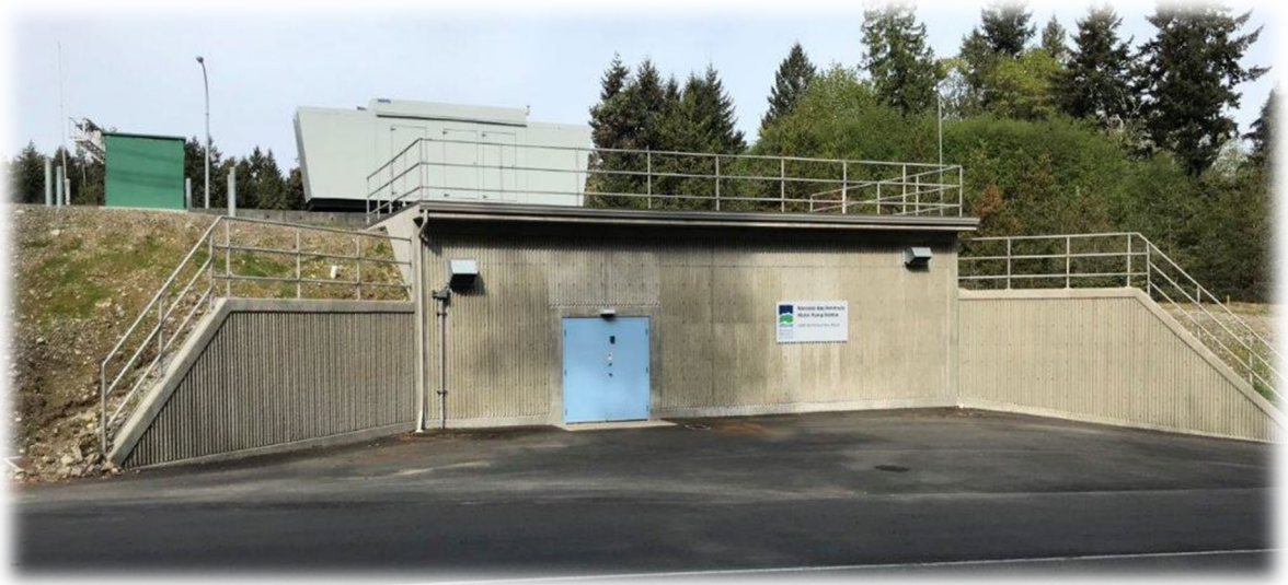
New Northwest Bay Road Pump Station (2019)
