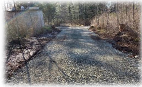
Tippet Road Well #1 Site (2022)
