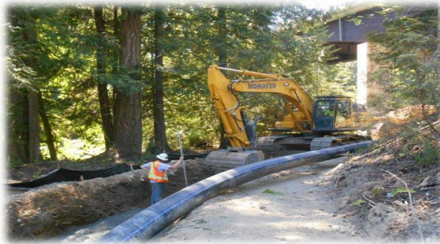
ERWS Bulk Water Transmission Line Construction near Hwy 19 (2017)
