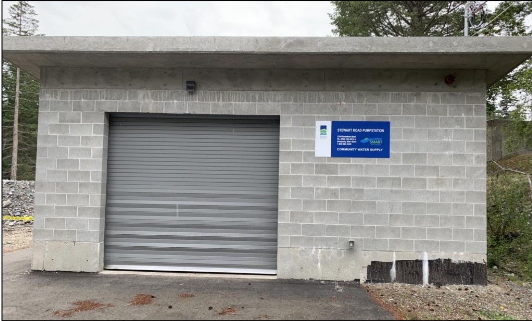
Stewart Road Pump Station (2020)
