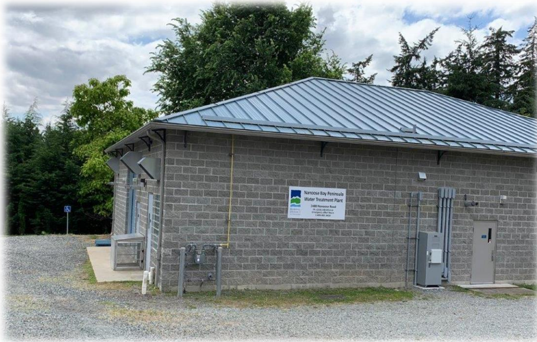
Nanoose Bay Water Treatment Plant
