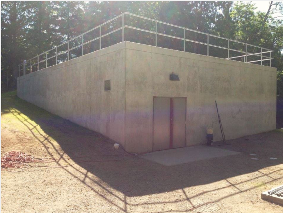
San Pareil Reservoir #2
