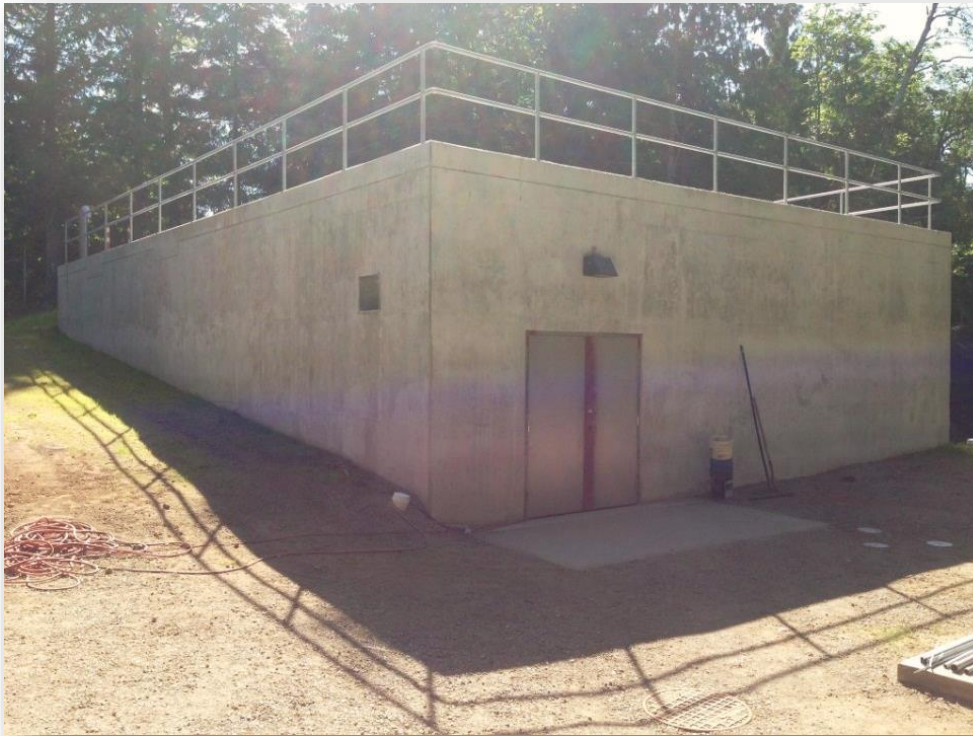
San Pareil Reservoir #2
