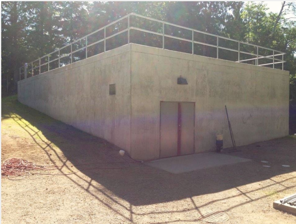
San Pareil Reservoir #2
