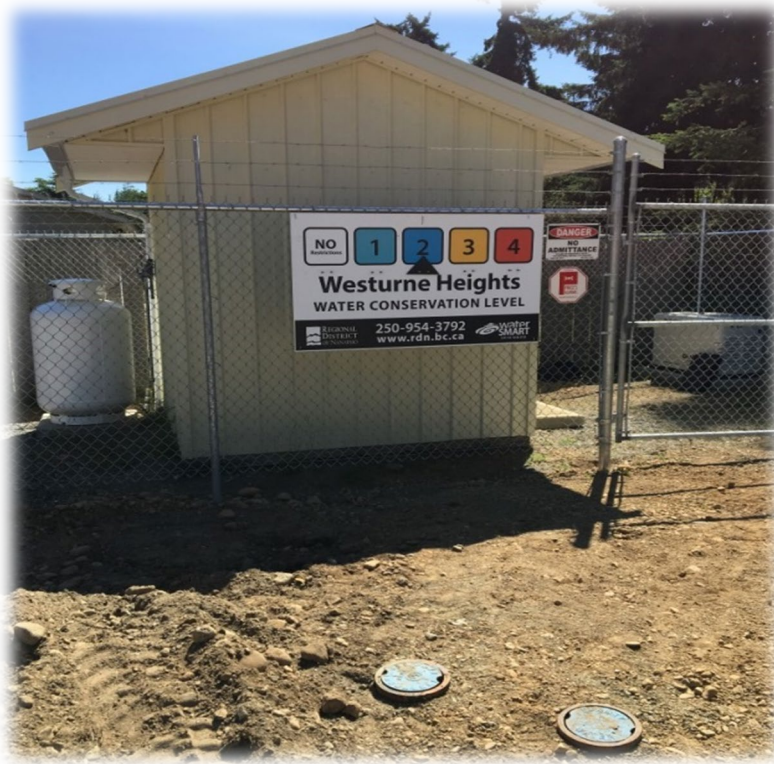
Westurne Heights Pumphouse and Buried Cisterns
