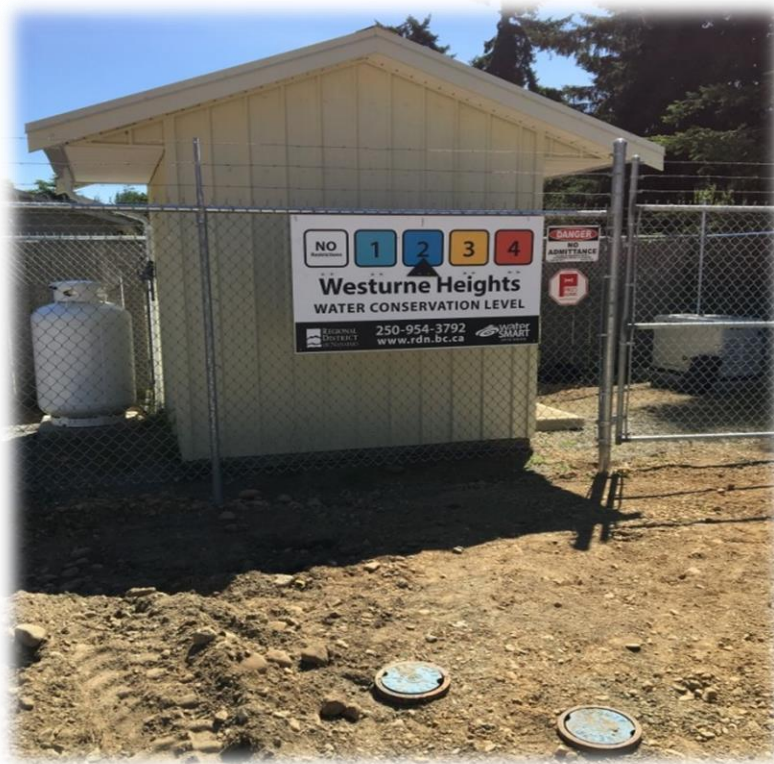
Westurne Heights Pumphouse and Buried Cisterns
