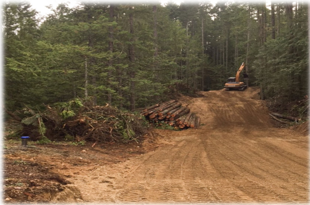
Land clearing and well site construction in Whiskey Creek
